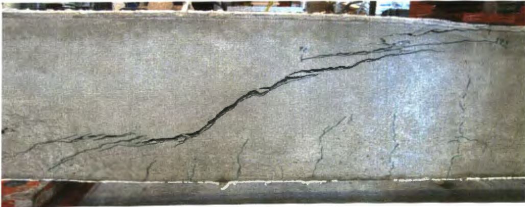
Figure 6.53. SCC-NS-2 Beam at Failure
