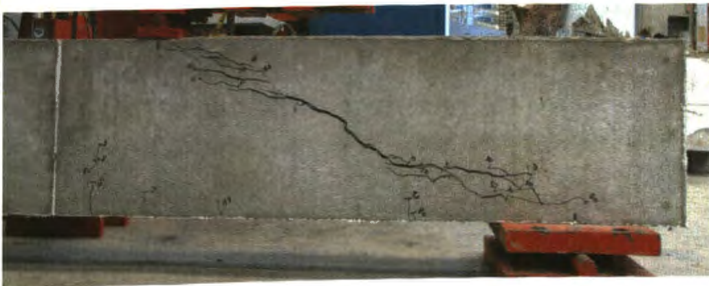
Figure 6.54. SCC-NS-3 Beam at Failure
