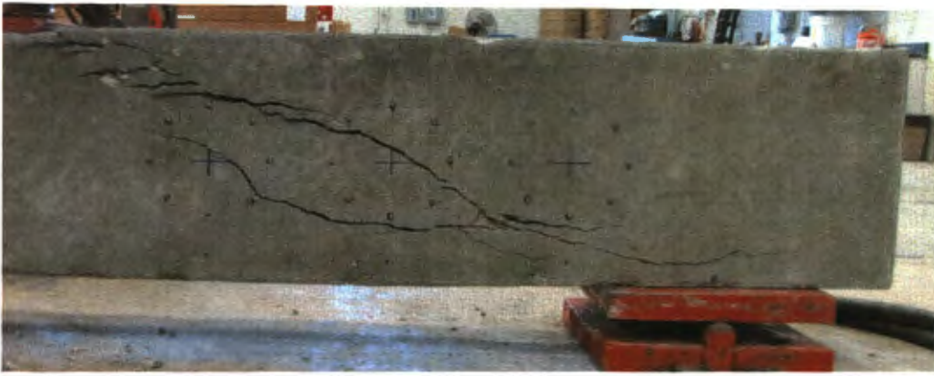
Figure 6.43. Control-NS-1 Beam at Failure
