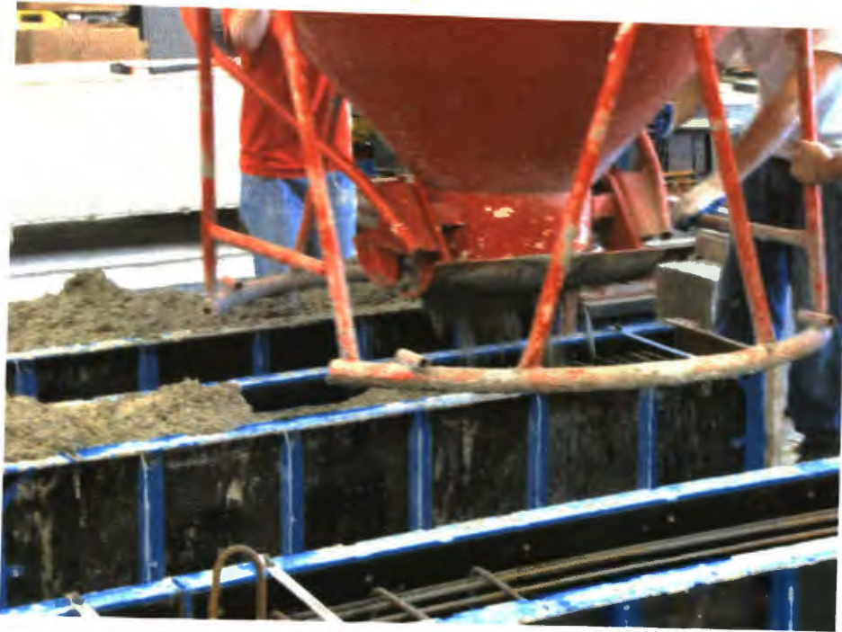
Figure 6.11. Placing Concrete
