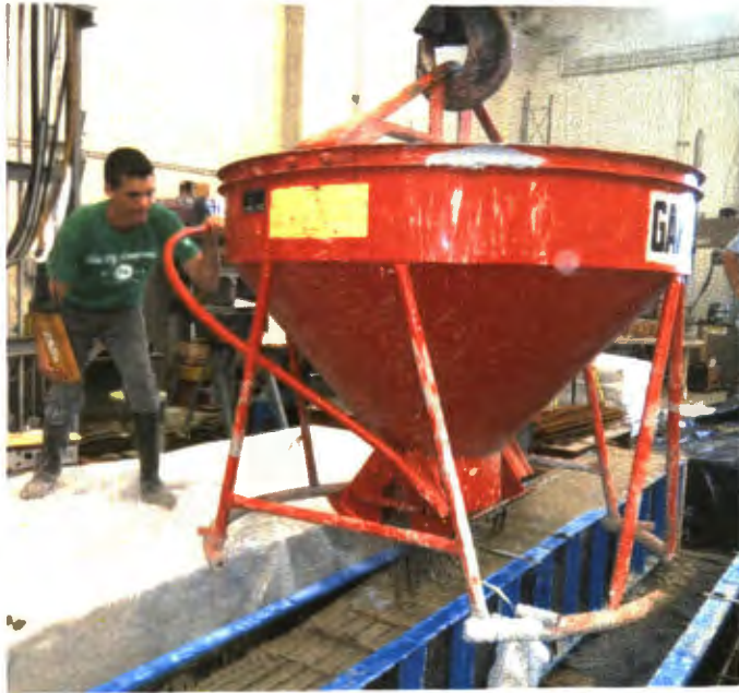
Figure 6.15. Placing SCC
