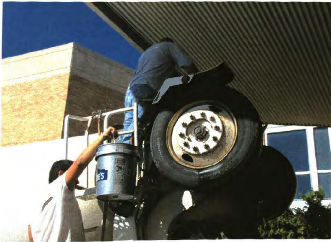
Figure 6.14. Addition of Chemical Admixtures
